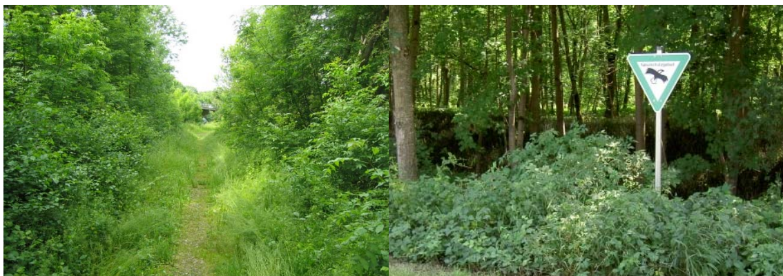
Figure 5: Extensive woody vegetation on levees on Bavaria (left: wooded dike at River Iller (Bavaria) near Altenstadt with a trail on dike crest, Source: TU Munich / right: complete wooded dike at River Danube near Dillingen in a nature protection area, Source: StMUGV, a ministry of Bavaria / both taken from Haselsteiner, 2019)
