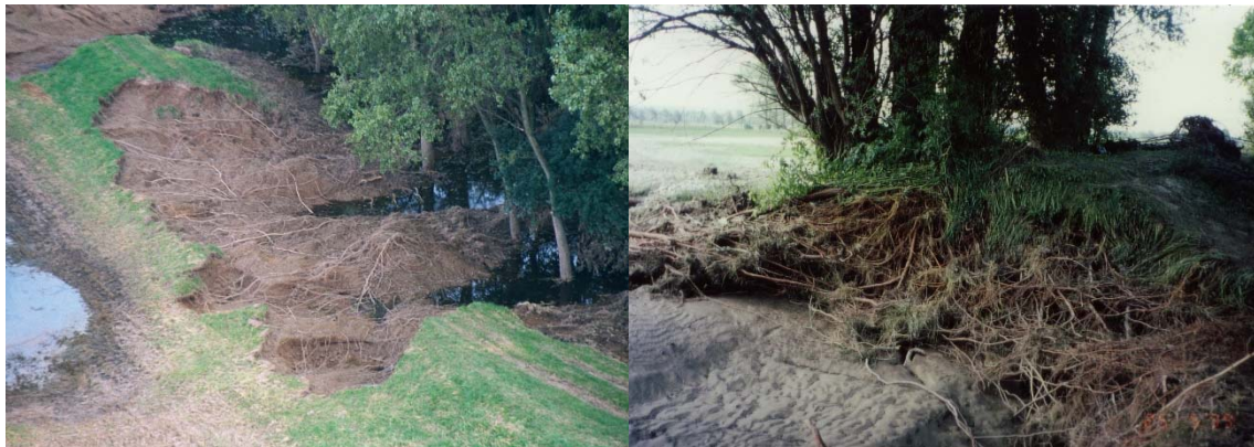
Figure 2: Roots through levees exhibited after dike breaches (left: failed dike at the River Mulde 2002, Source: Landestalsperrenverwaltung Sachsen / right: dike breach at the River Ammer in Bavaria in 1999, Source: WWA Weilheim)
