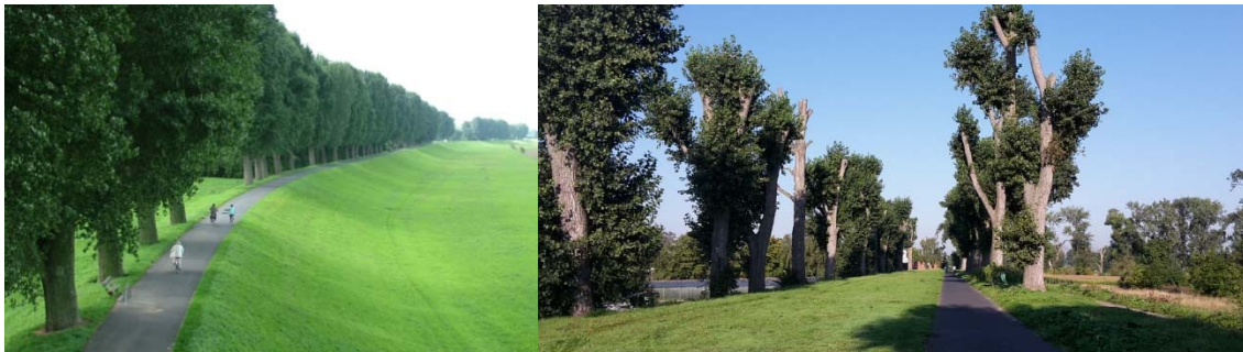
Figure 9: Trees on levees within the vicinity of the town Duesseldorf at the River Rhine (left: row of poplars on the crest of the “Lohausen” levee in Duesseldorf, Source: Bezirksregierung Duesseldorf / right: poplars on the relatively wide-crested “Niederkasseler” levee in Duesseldorf – 2015, Source: BCE)
