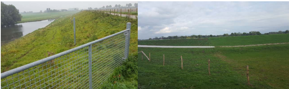
Figure 3: Vegetation layers in form of grass covers of selected case studies (left: upstream slope of Rhine main levee in 2017 with sheep herd in the back / right: downstream slope of a Rhine levee showing different management/cultivation measures from 2019 / Source: BCE)
