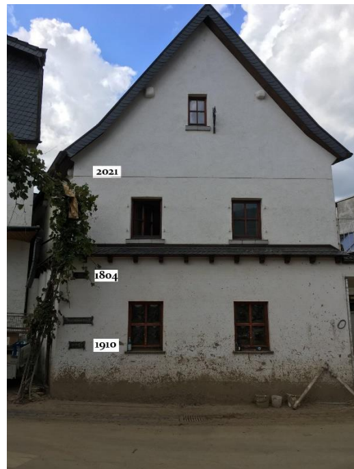
Picture 5: Flood marks at a house in the village Dernau (Source: Mr. Matthias Habel, see also Roggenkamp, 2021)
