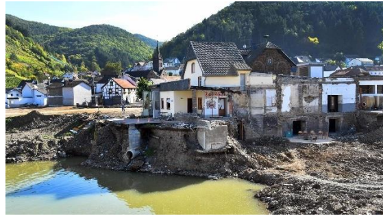
Picture 4: Erosion and destruction of houses in the village Dernau (Source: www.deutschlandfunkkultur.de )
