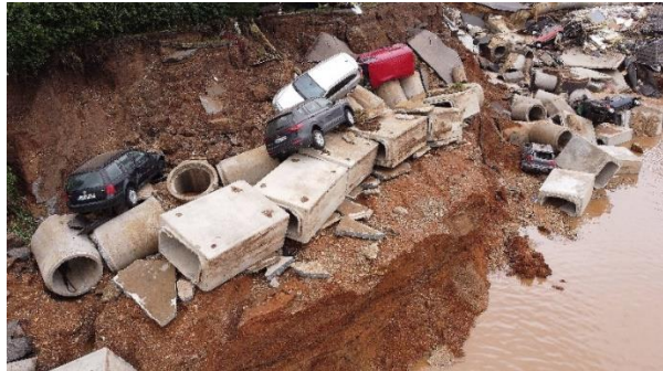
Picture 2: Flood damage in Erfstadt Blessem (Source: https://rp-online.de/ )
