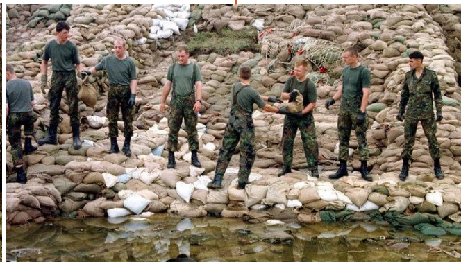
Levee defence works carried out by soldiers during Oder flood 1997 (Source: www.planet-wissen.de)
