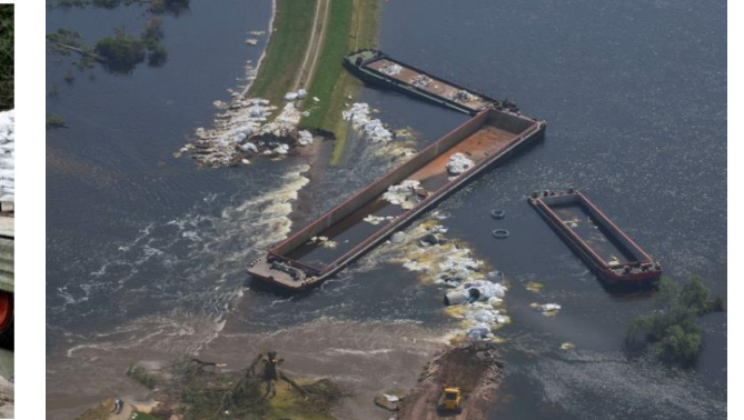
Elbe Flood 2013 – Levee failure near the village Fischbeck, Source: Jüpner (2016)
