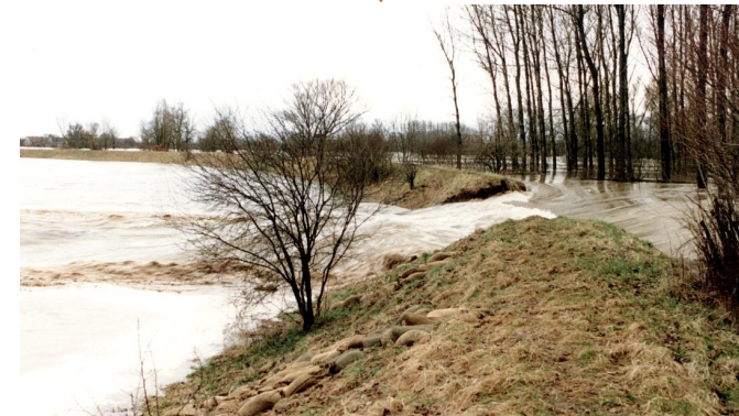
Levee failure nearby Stadldorf during Danube flood 1988 – initial breachign stage, Source: WWA Deggendorf
