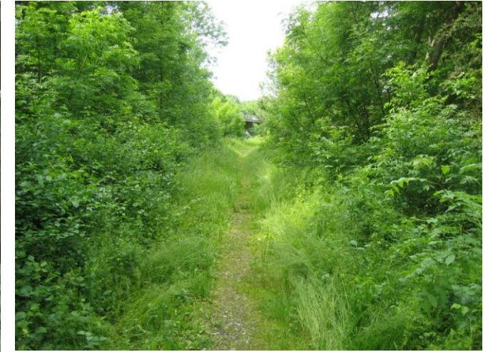
Wooded levee at the River Iller nearby Altenstadt (Source: TUM)
