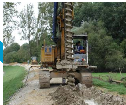
Bored pile wall in dike at River Danube (Source: WWA Ingolstadt)
