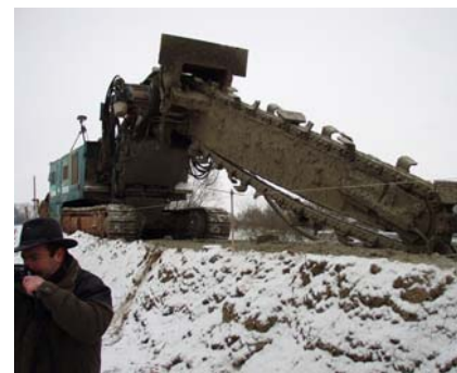
Milled cut off wall in dike at River Danube (Source: TUM)
