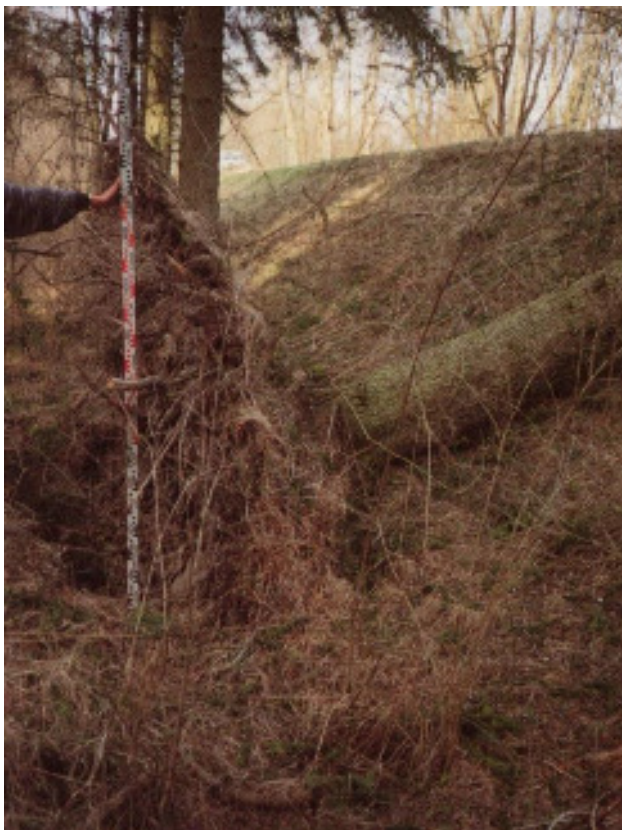
Thrown spruce at the landside dyke toe at the river Lech (taken from LfW BY 1990)
