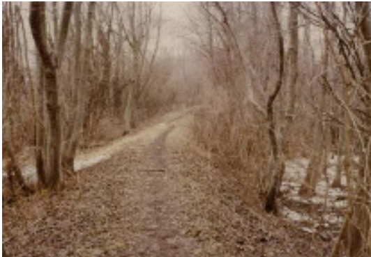
Flood protection dike at the River Ammer (year 1979; Source: WWA Weilheim)
