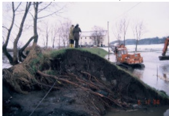
Dike breach during flood incident 1988 at Höselhurst in Danube (Source: TUM)
