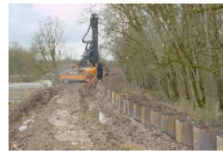
Sheet pile wall in dike at River Danube (Source: WWA Ingolstadt)
