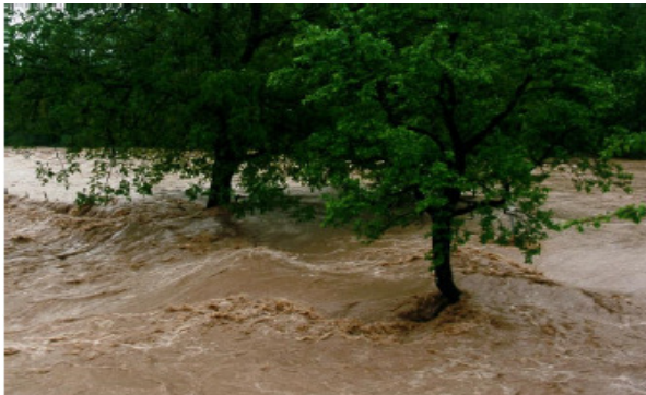
Breakage of Loisach dike in Bavaria during the Spring flood 1999 (Source: WWA Weilheim)
