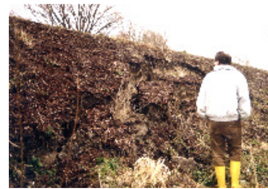
Sliding of top soil layer at the landside slope at river Danube 1988 (Source: WWA Deggendorf)
