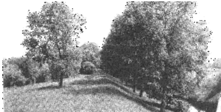
Flood protection dike at the river Koeßnach near with poplars and meadow (year 1985, taken from Hacker et al. 1999)
