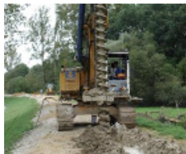
Bored MIP wall in dike at River Danube (Source: WWA Ingolstadt)
