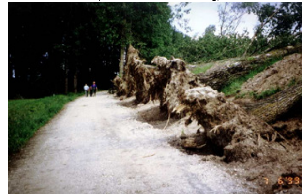
Tree failure at a dike in Germany 1999 (Source: StMUVG NRW)
