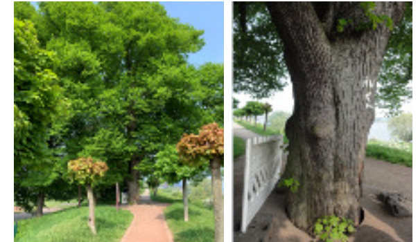
Flood protection dike at the river Rhine, Orsoy, tree on dike crest (Source: BCE, 2019)
