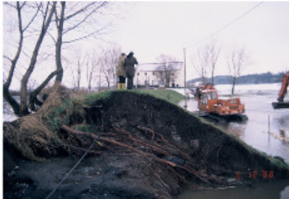
Breakage of the dike near Höselhurst on the Danube during flooding 1988 (Source: TU Munich)
