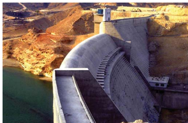
Figure 5. View of Dayqah Dam from the left abutment (taken from RMD, 2014).
