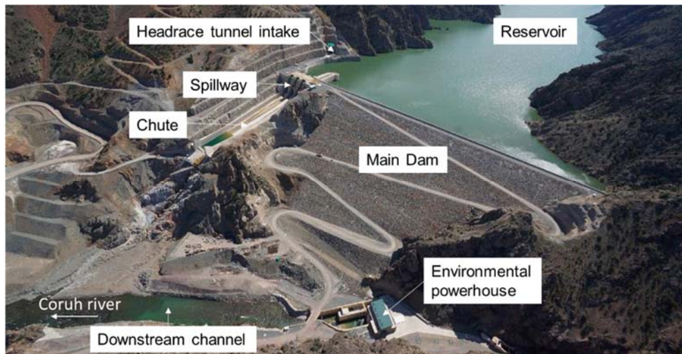
Fig. 2. Downstream view of the main dam with environmental powerhouse on the right side of the picture (Source: EnerjiSA)
